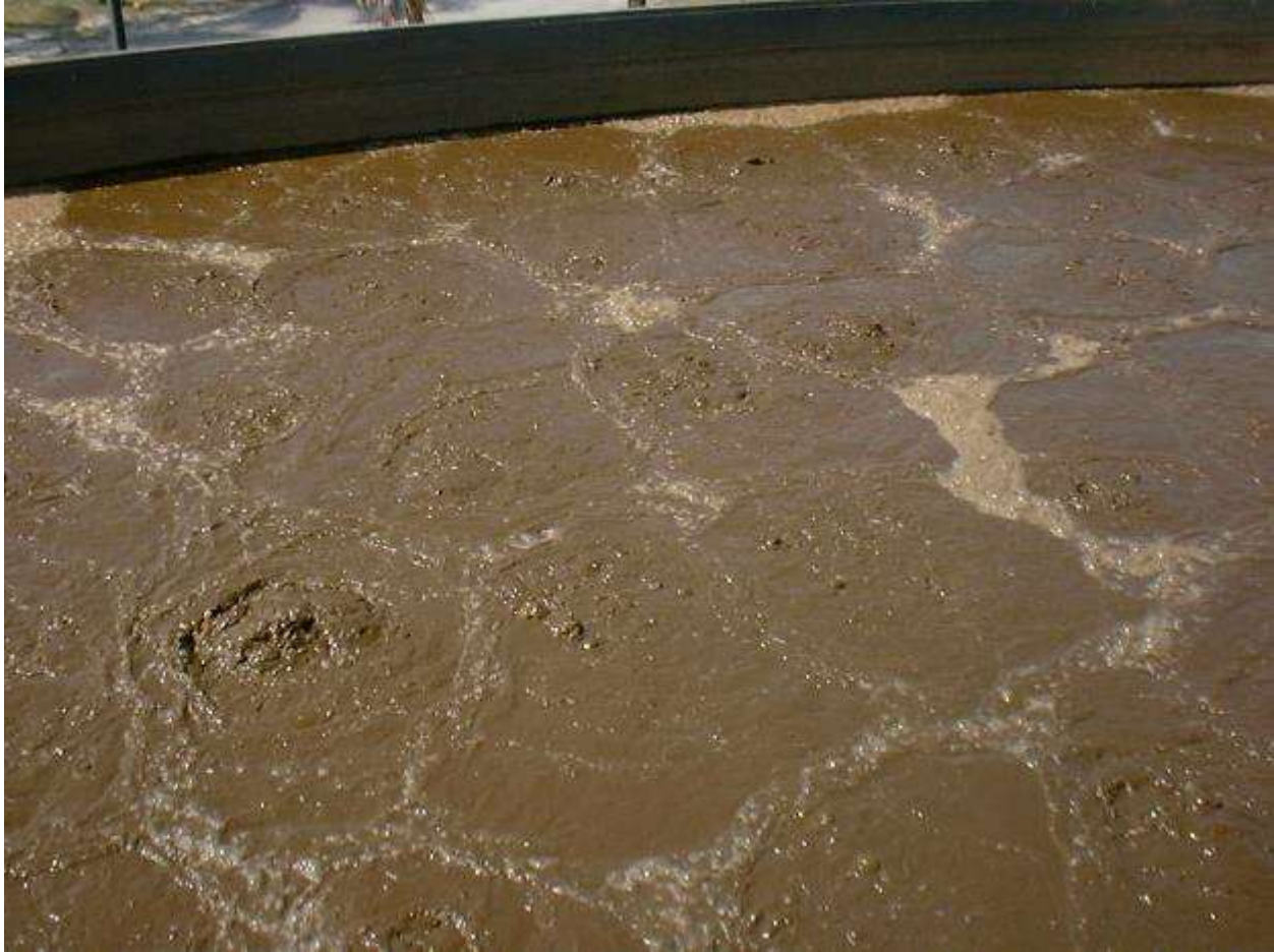
Figure 14. Activated sludge process
