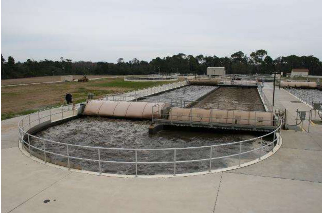
Figure 17. Extended aeration basin
