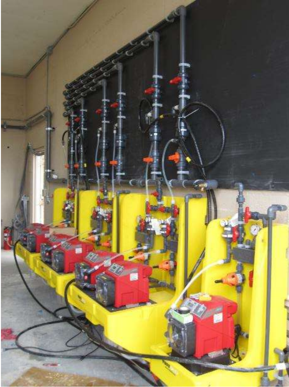
Figure 21. Chlorinator equipment
