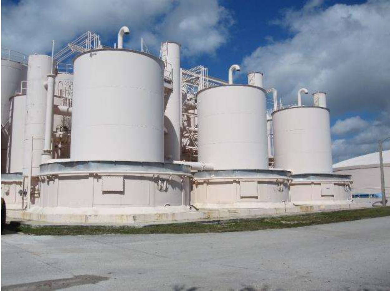
Figure 24. Pressure filters
