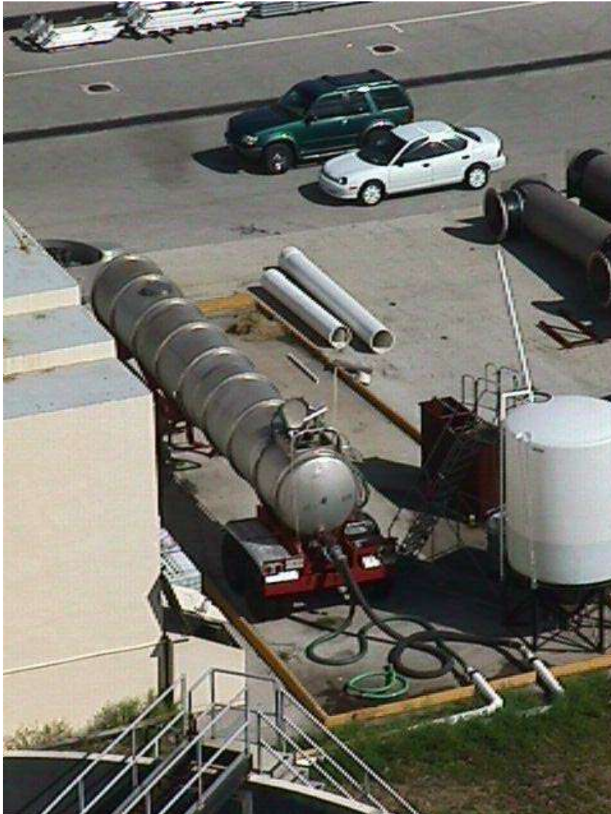
Figure 10. Electron beam treatment unit at the Central District WWTP (Slifko 5/10/18 presentation at Fermilab)
