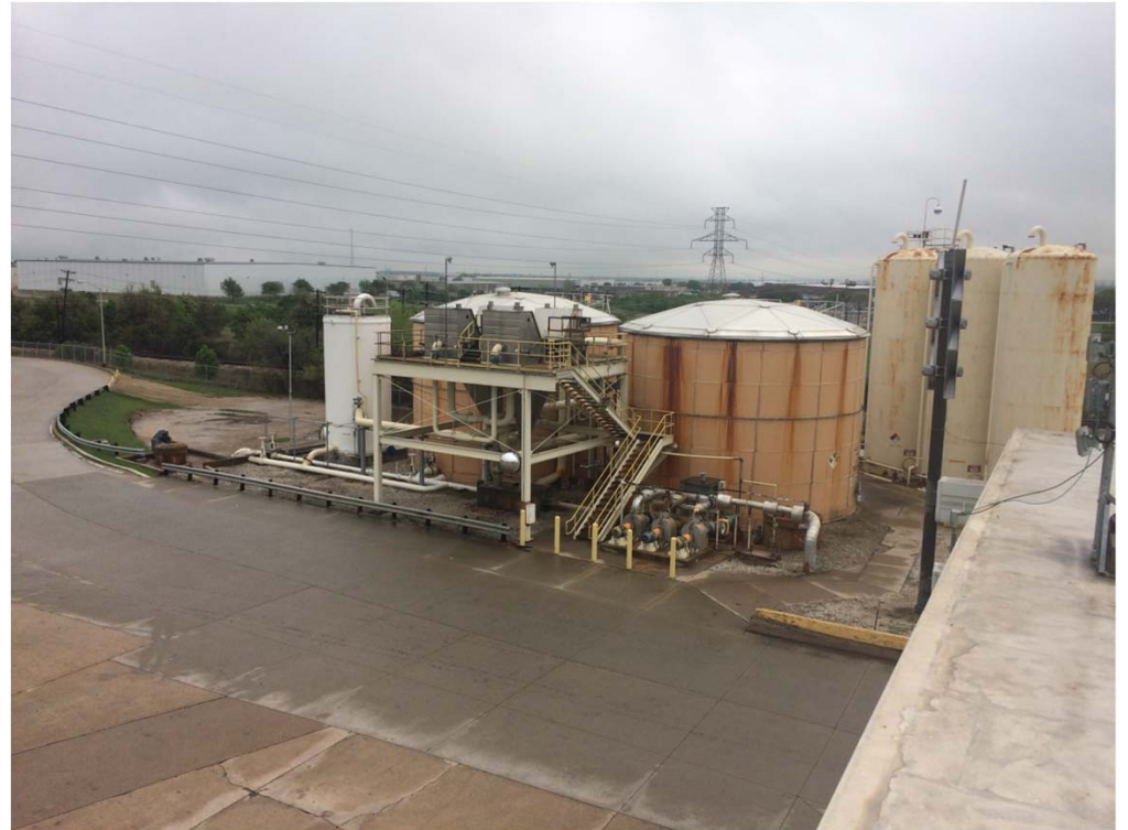
Fort Worth wastewater treatment
