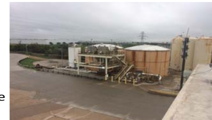
Fort Worth wastewater treatment
